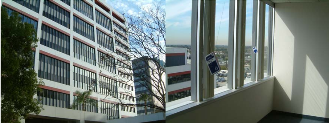
Figure 6 Film applied south facing 8 th floor
